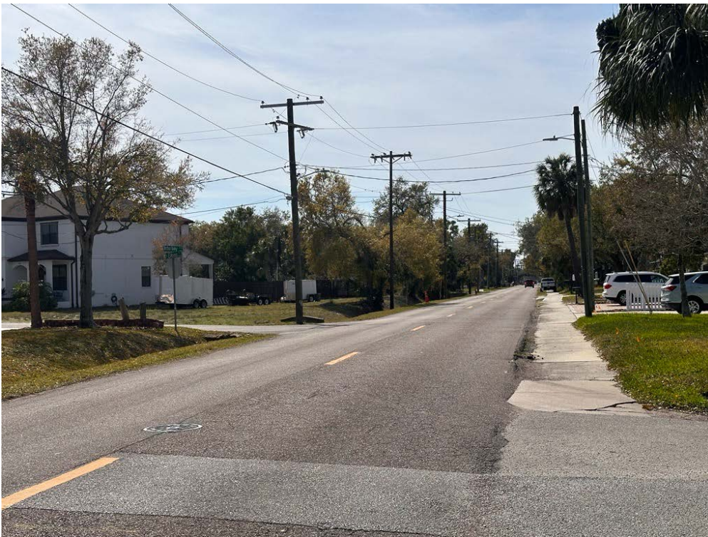
Photo 3-3. Sidewalk without Protection from Vehicles and with Minimal Tree Canopy in South of Gandy
