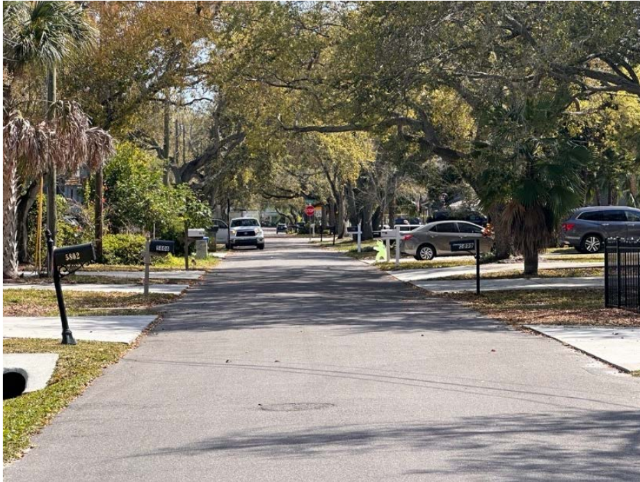
Photo 3-1. South of Gandy Neighborhood Road without Sidewalk and Open Drainage
