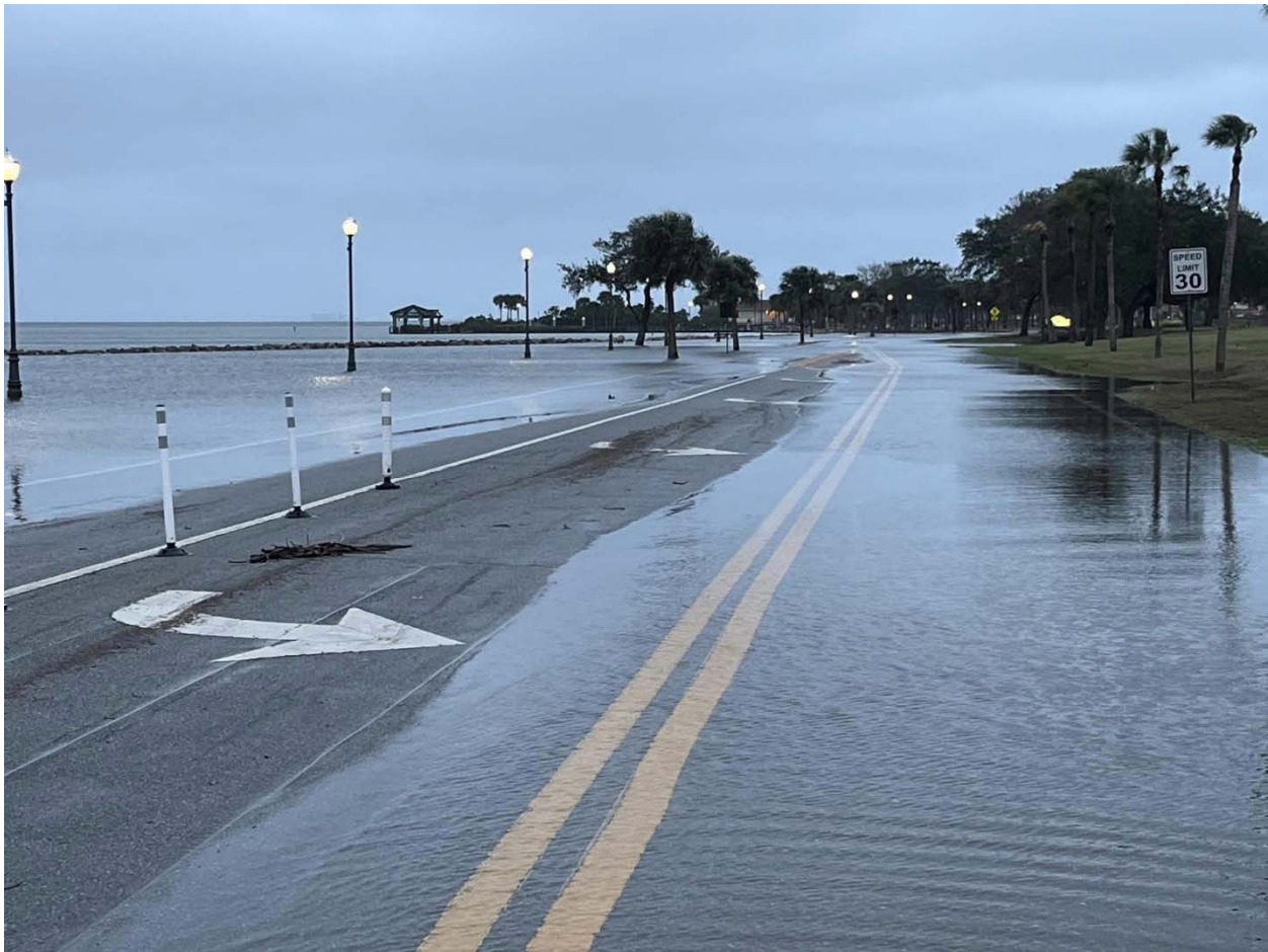
Picture 3-5. Coastal Flooding along Bayshore Boulevard
